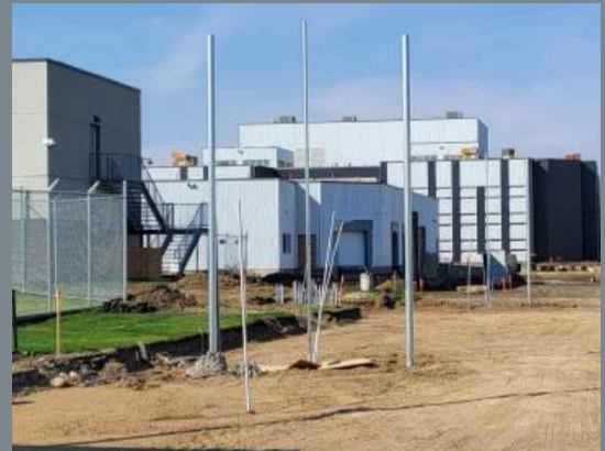
Saskatoon Provincial Correctional Centre
